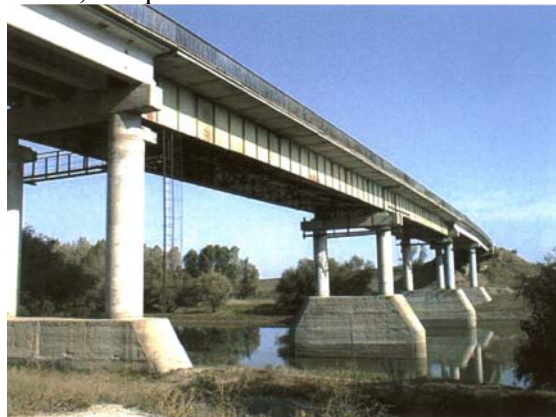
Picture 1. General view of the bridge from the right bank of the river
