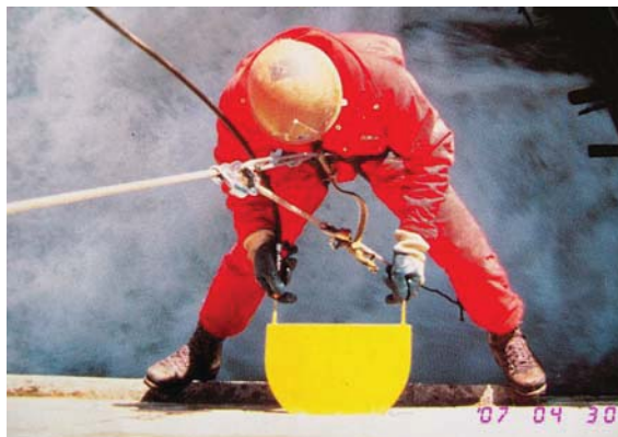
Fig.5. Survey to perform flat-jacks test
