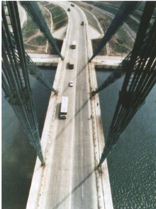
Figure 1. The Agigea Bridge from Romania
