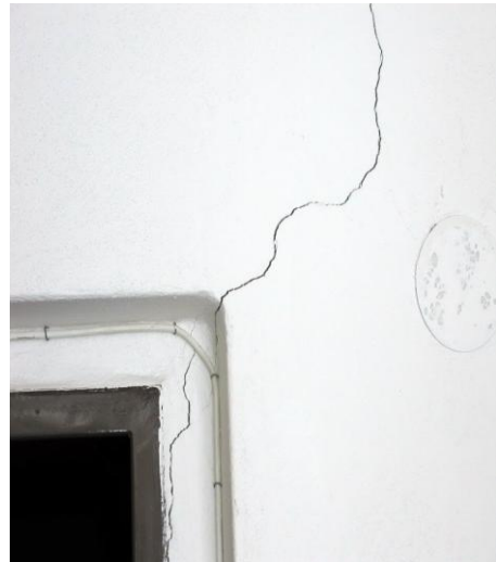
Figure 2. Cracking in the brickwork
