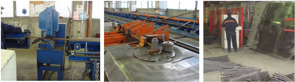
Fig.2.3. (a) cutting, (b) shaping, (c) building the stirrups
