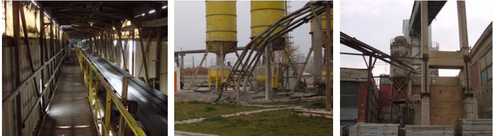
Fig.2.5. (a) conveyor belt, (b) cement pipes for transport, (c) station for concrete preparation
