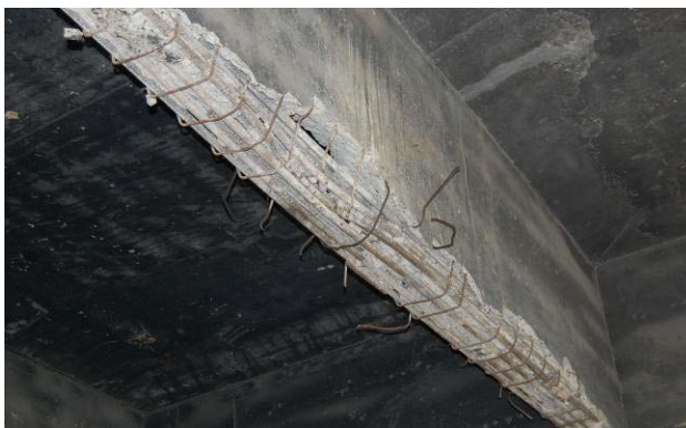
Figure 4. Beam 2 (central beam)
