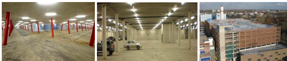
Figure 17. Parking places made with concrete slab with spherical gaps system
