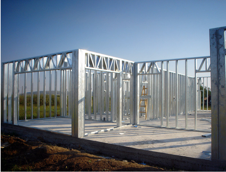
Figure 1. Structure made of light-gauge steel profiles
