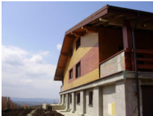
Figure 1. Frontal view of the south façade
