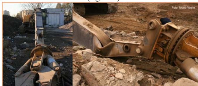
Figure 5. Hydraulic scissors arm of 21 m damaged
