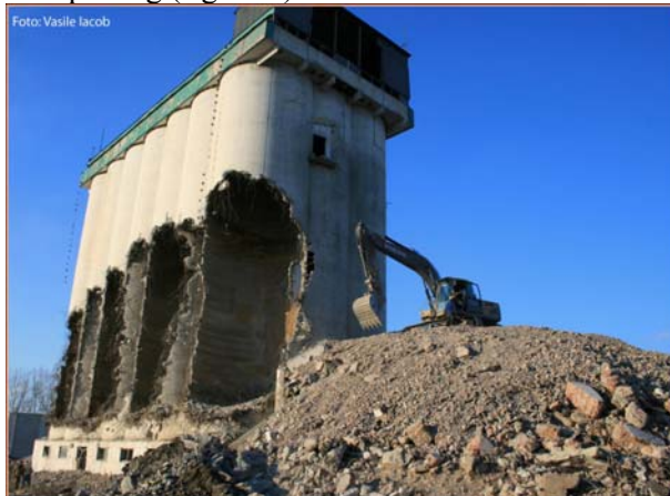
Figure 6. Arranging ramp access to the objective to be demolished
