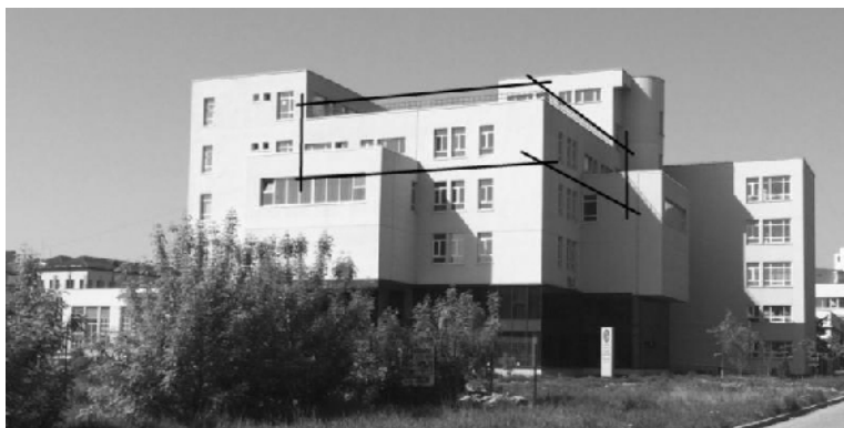
Figure 1. Building used for analysis
