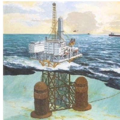
Figure 2. Maureen steel gravity-based platform, U.K.
